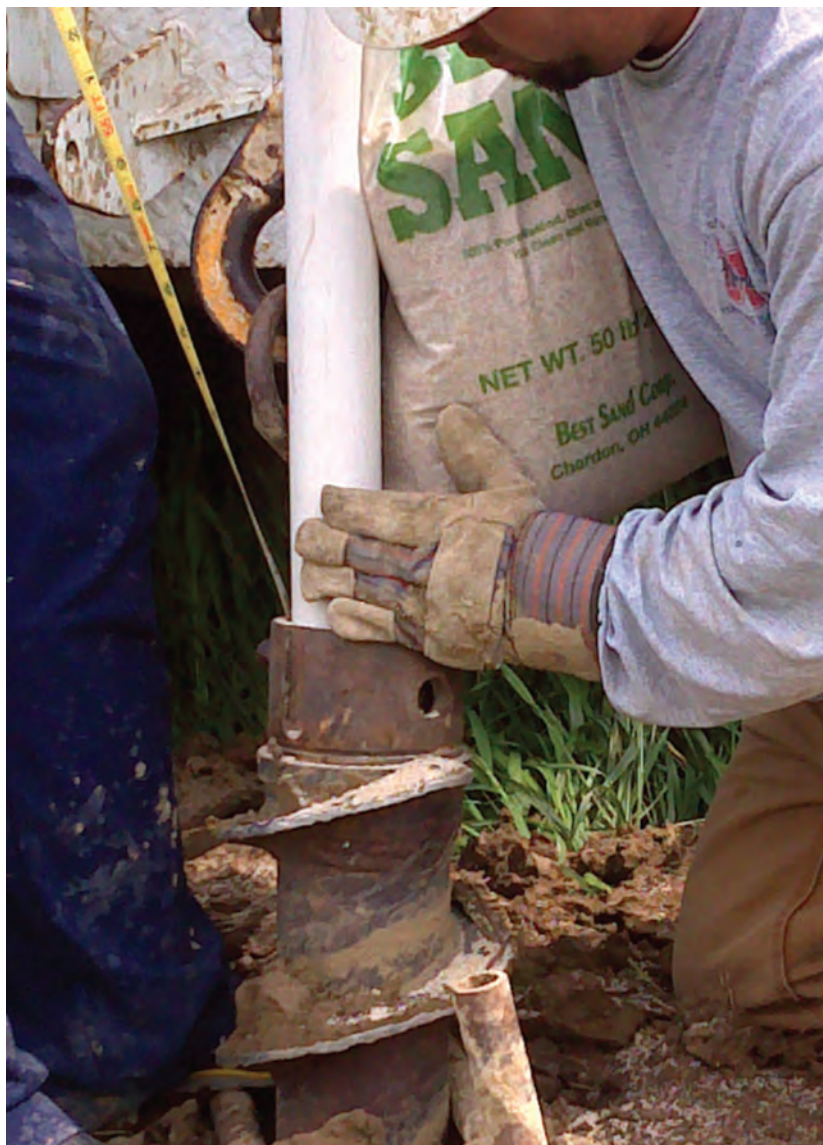
University of Nebraska Conservation and Survey Division staff installing a monitoring well near Clearwater, NE.
